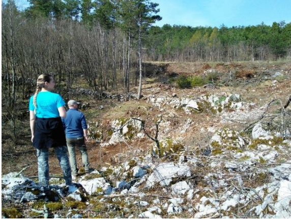
Photo 1. Visit at the railway construction site (photo M. Aljančič).
